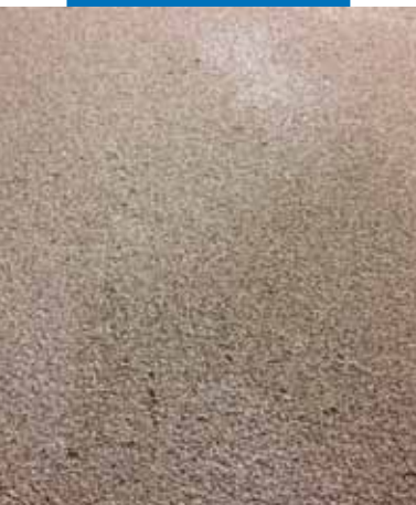
Compact method- basecoat scattered Mapequartz color
