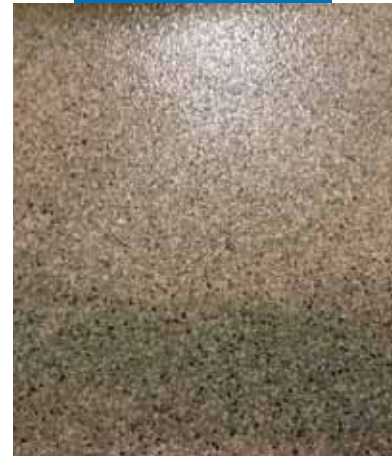
Compact method - finished floor
