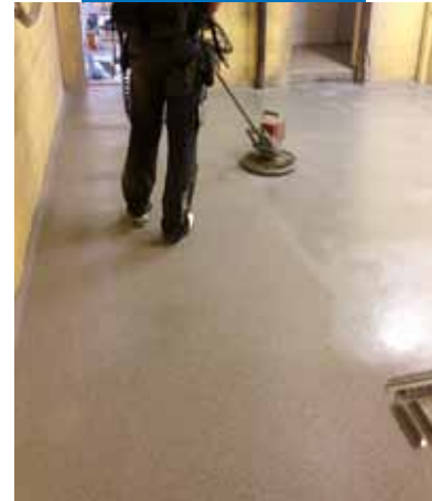
Compact method - compacting with power trowel
